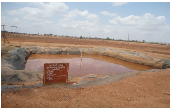
Figure 12: Farm pond lined with Soil: Cement (6:1).
